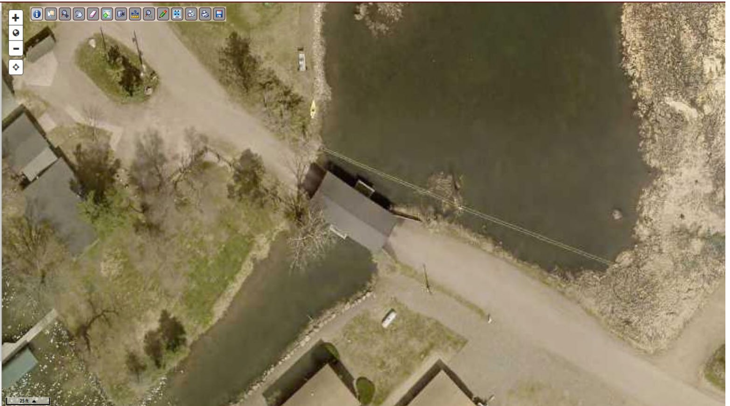
Crossing area prior to construction.
